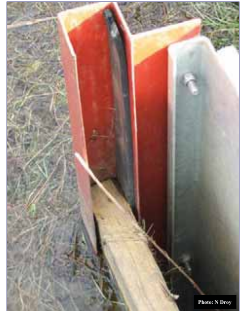
Fig 5: Detail of rubber seal on structure
