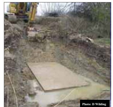
Fig 2: Concrete pad for base
