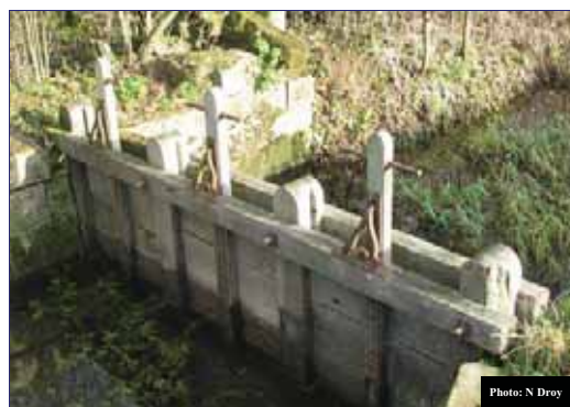
Fig 5: A traditional wooden penstock weir
