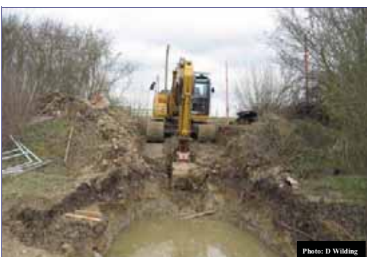
Fig 3: Installation of tilting weir
