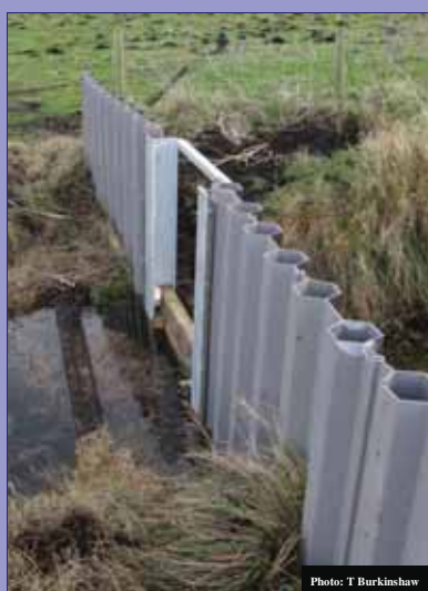
Photo: T Burkinshaw
