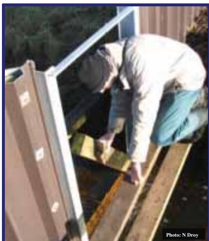
Fig 3: Inserting a dropboard
