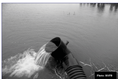
Fig 4: Water flowing through control pipe
