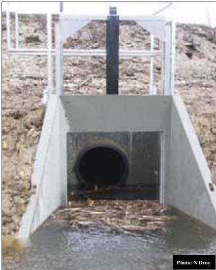
Fig 1: Overflow weir
