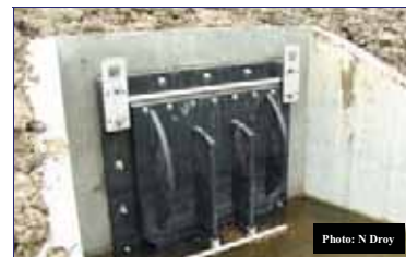
Fig 4: non-return flat valve
