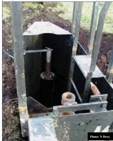
Fig 2: Custom made trenching box
