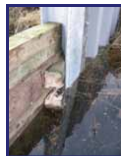
Fig 2: Dropboards and wooden chocks
