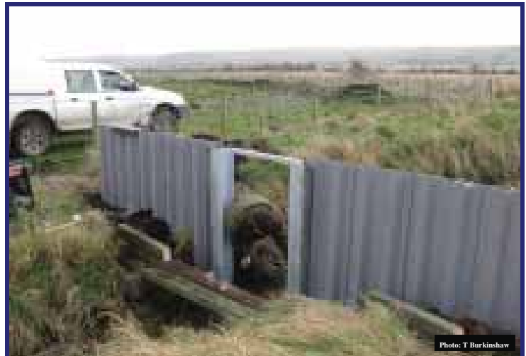
Fig 4: Installation of sluice
