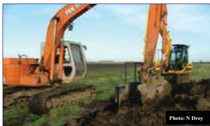
Fig 1: Installation of plastic sheeting
