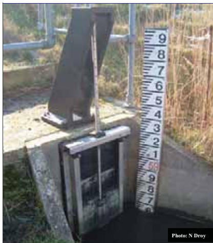
Fig 1: Penstock weir & gauge board
