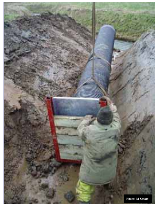
Fig 3: Lowering the sluice unit in to position
