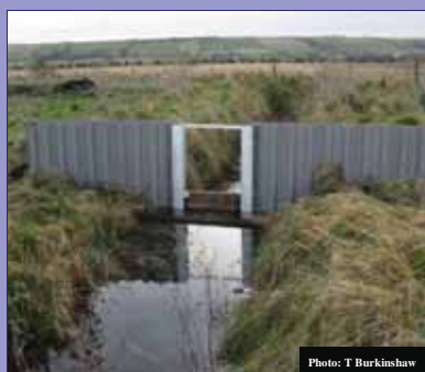
Photo: T Burkinshaw
