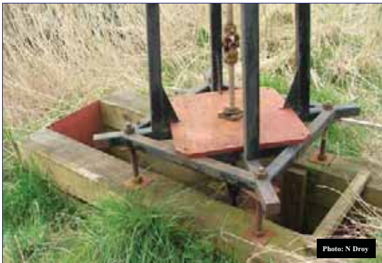
Fig 5: Sail unit is secured to pumping chamber
