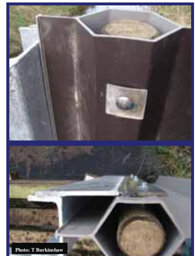
Fig 6: Sluice frame & wooden supports
