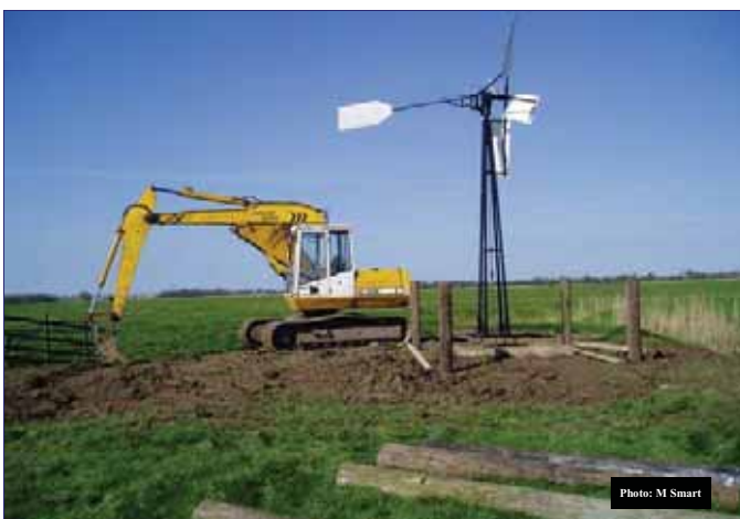
Fig 4: Installation was completed within one day
