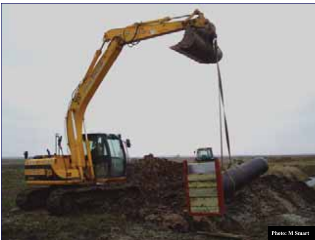
Fig 2: 360 excavator installing sluice structure
