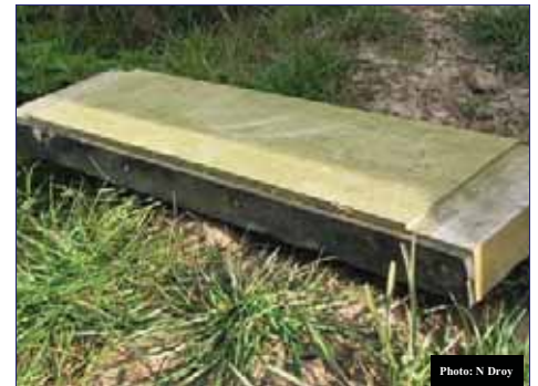
Fig 6: Drop board with rubber seal
